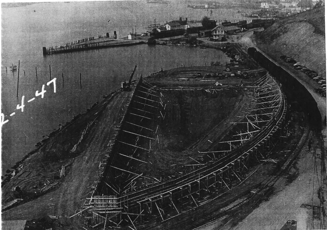
Figure 13: Feed Warehouse construction, 19 February 1947, 4 February 1947, Vallejo Historical and Maritime Museum Collection.
