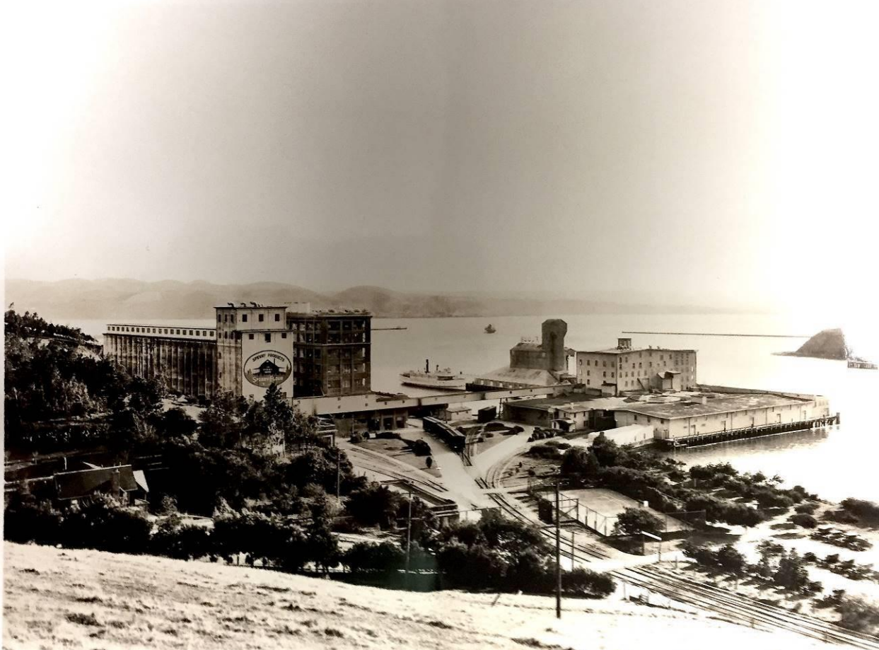
Figure 11: Sperry Flour Mill from hillside with Manager's Residence lower left, Grain Elevator and Mill center left with rooftop garden visible atop mill building, and tennis courts lower right, 1935, Vallejo Historical and Maritime Museum Collection.
