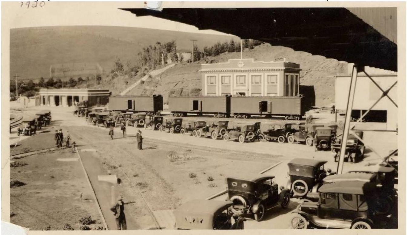
Figure 10: Sperry Flour Mill from under the conveyor bridge with Administration and Laboratory Building center frame behind railroad cars, Manager's Residence on the hill, and Company Garage left, 1920, Vallejo Historical and Maritime Museum Collection.
